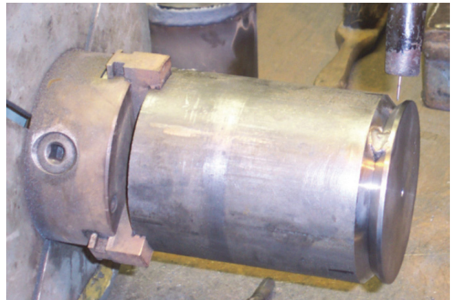
Steel tube and Dura-Bar Butt Plate, bevel & socket joint, ready for welding
